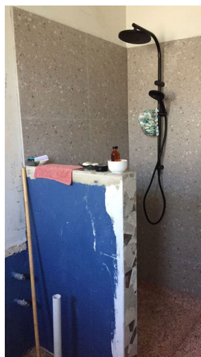
Construction progress shot.
